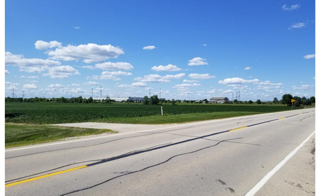
The existing roadway is generally one lane in each direction with paved or gravel shoulders. Grass ditches drain the roadway. This is commonly referred to as a rural cross section.
